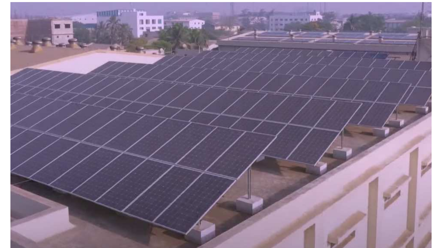
Project Surbhi Mills by Goldi Solar
