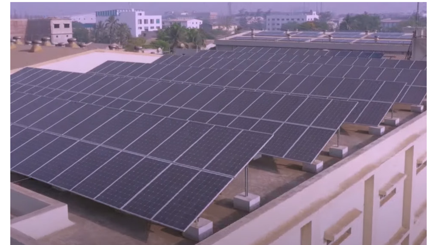
Project Surbhi Mills by Goldi Solar
